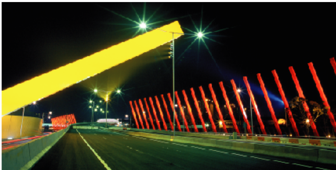
WESTERN LINK FREEWAY ART FORM LIT WITH DICHROIC YELLOW #7001
